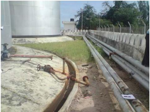
Tank farm at GAPCO Oil Company. The valve and pip on the left is used to drain seawater from the tank.
