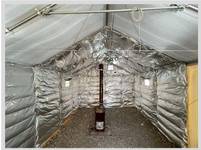
Figure 3: Recycled PP plastic waste encapsulated in tarpaulin panels for insulation.
