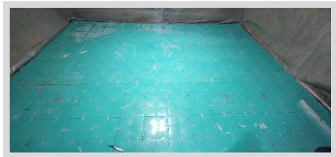
Figure 4: PP plastic waste is recycled into floor tiles.
