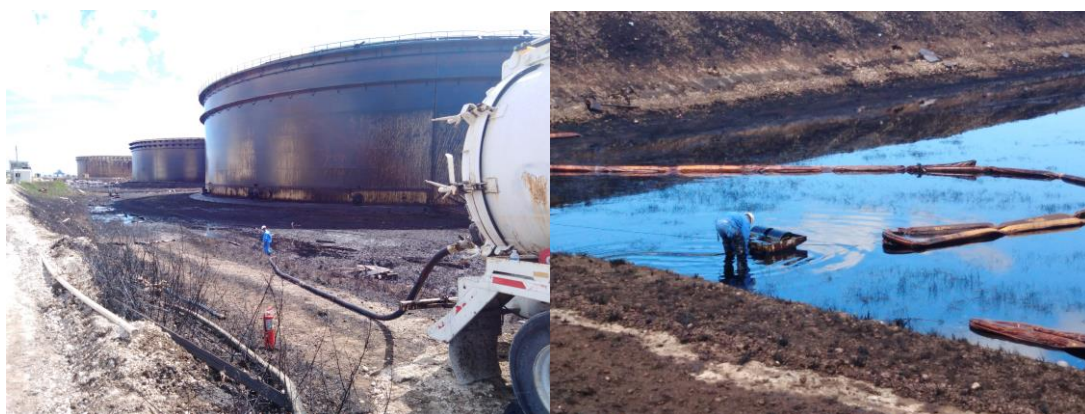
Figure 10 (left) and 11 (right): Collection of crude oil is carried out using vacuum trucks (left) and oil skimmers (right)
