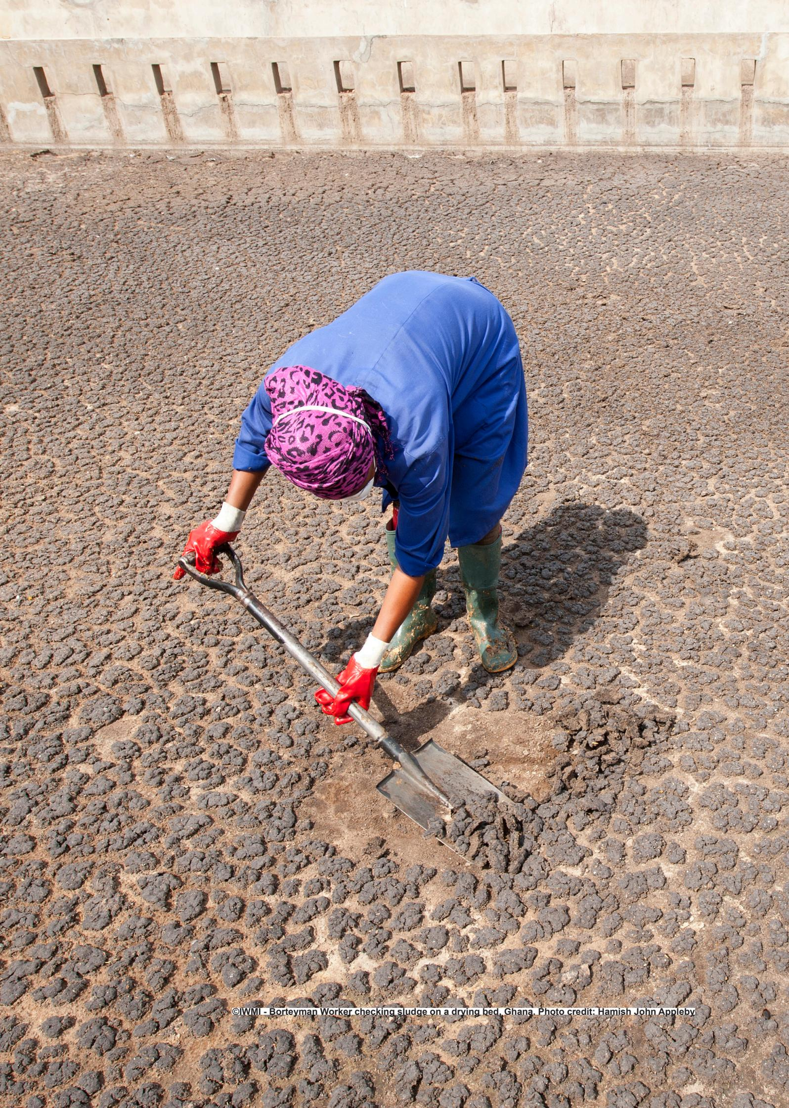
©IWMI - Borteyman Worker checking sludge on a drying bed, Ghana. Photo credit: Hamish John Appleby
