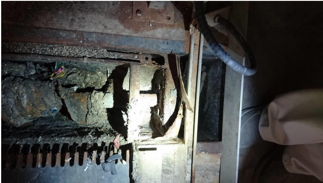
Picture 5: Roseau wastewater filtering station, first screening level, and broken endless screw used to compact the extracted material. 13.10.17 Ncl
