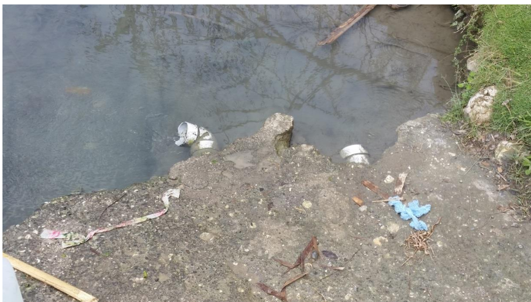
Picture 3. Broken and obstructed pipes at the Rosier water catchment, Roche-a-Bateau, Haiti @Eva Andersson
