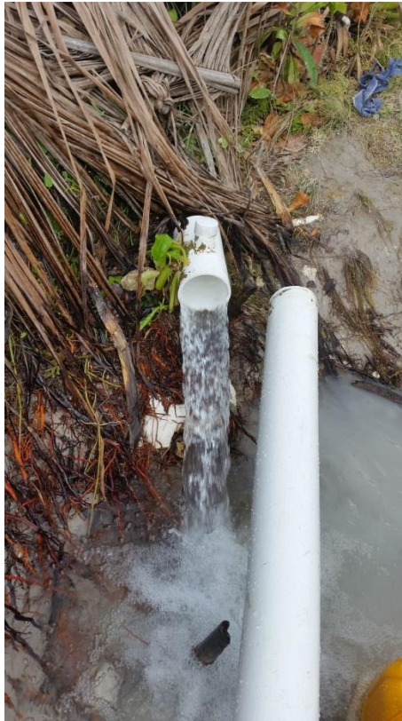
Picture 2. Broken pipes after Hurricane Matthew, Cascade, Port-Salut, Haiti @Eva Andersson
