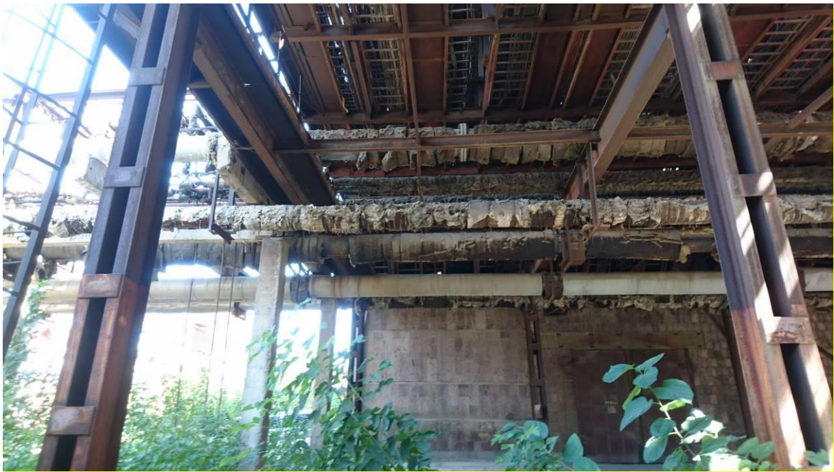
Picture 18: The lowest pipe is covered with a fibered cement potentially containing asbestos, the other pipes seem to be covered with glass wool material. (Sept 2017)
