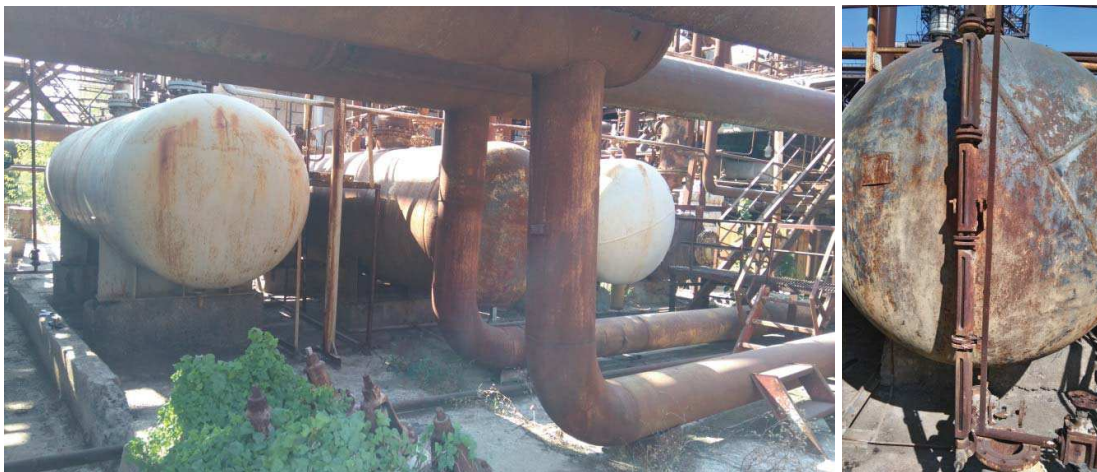
Tanks exposed to weather conditions presenting signs of corrosion
