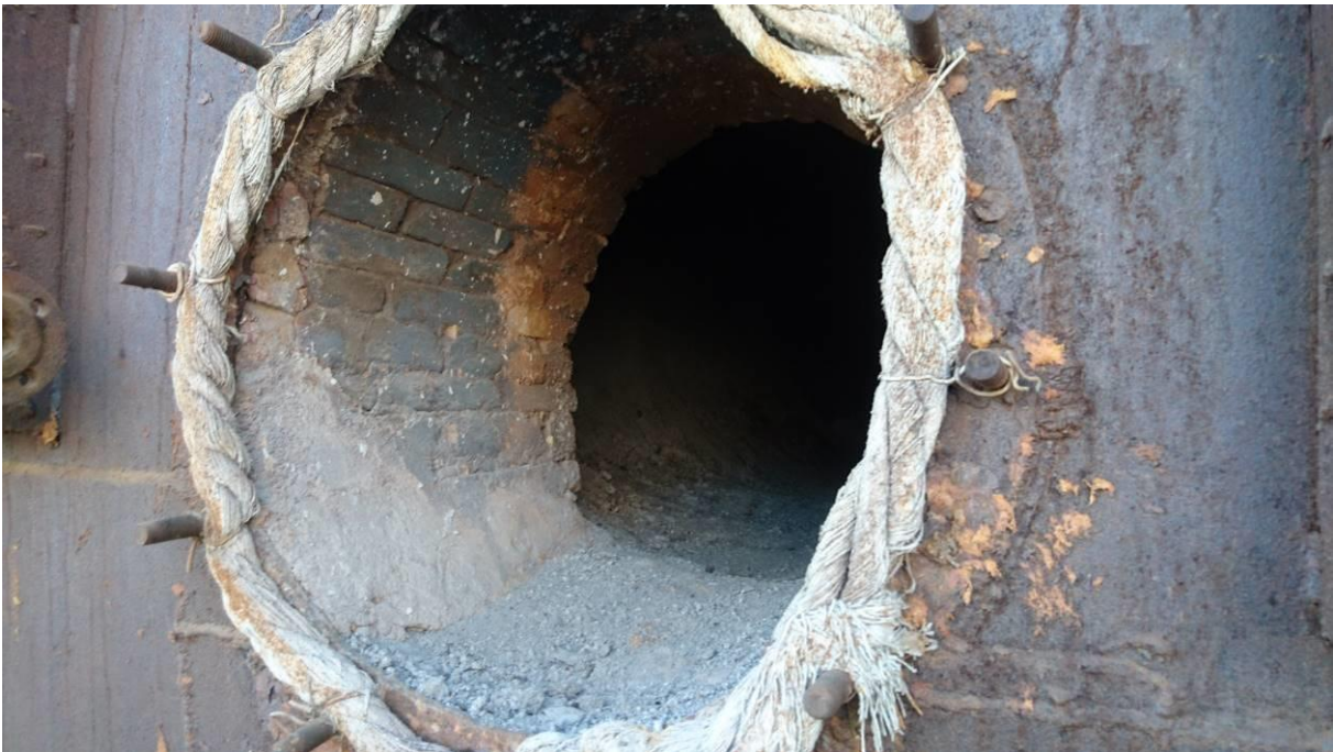
Picture 16: Potentially containing asbestos seal (Sept 2017)
