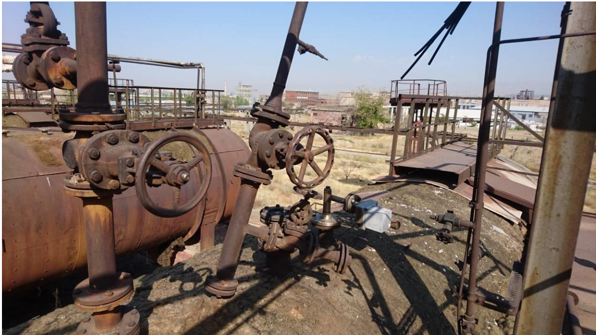
Picture 27: Storage 15, valves are blocked....
