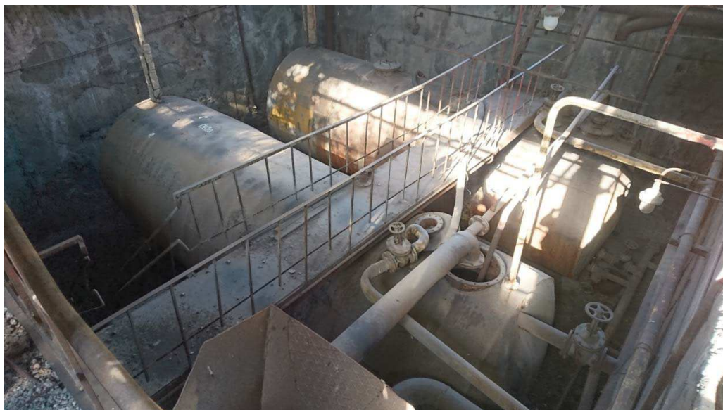
Tanks located below ground level, in an concrete pool
