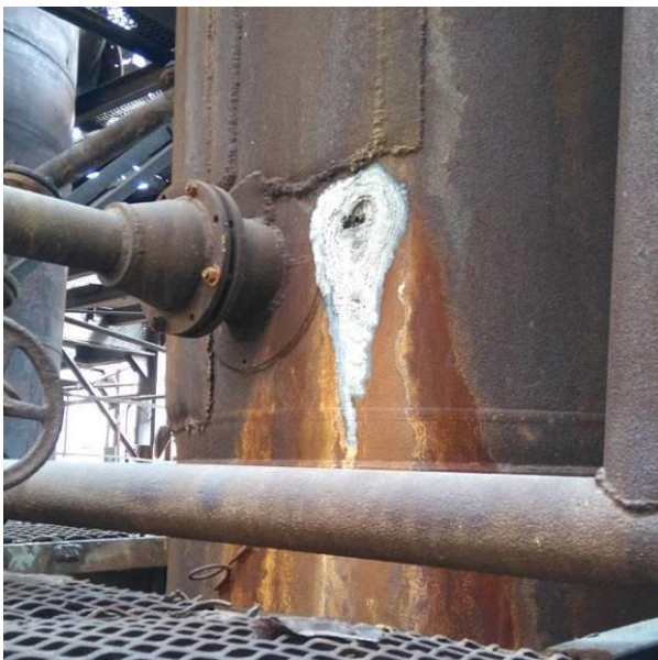
Picture 22: Old leak due to corrosion on acid tank
