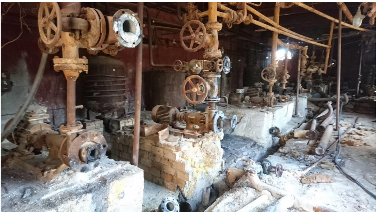
Picture 12: Sulfuric acid pumping station being dismantled (Sept. 2017)
