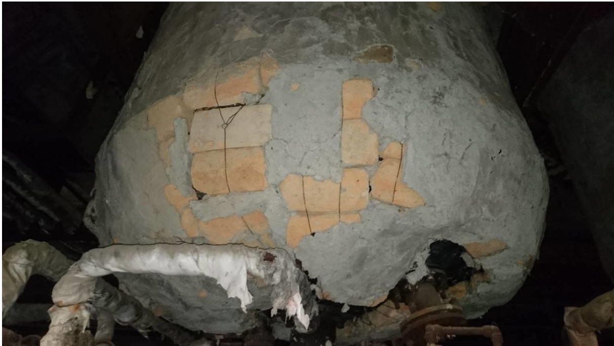
Picture 19: Reactor insulation potentially containing asbestos
