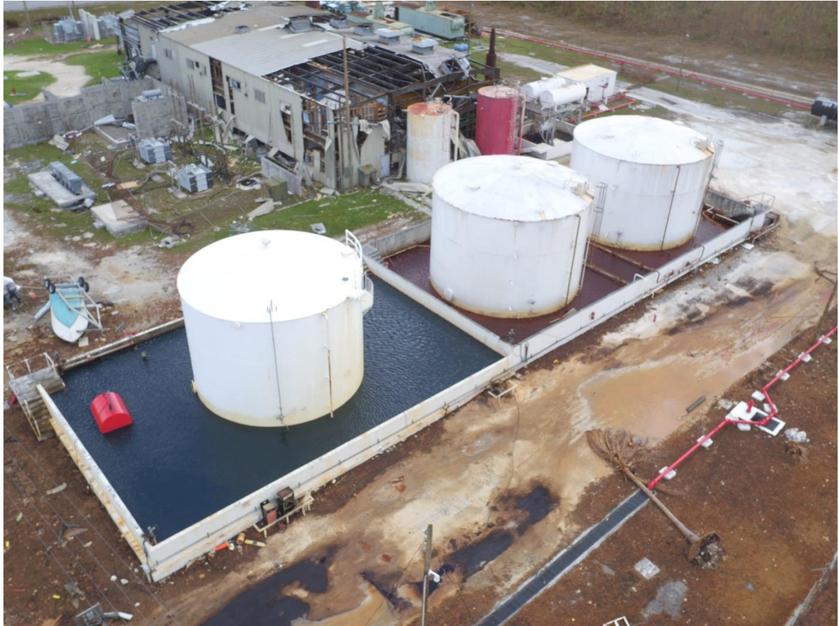
Figure 3: drone view of BPL Marsh Harbour power sub-station, showing the three tanks, the amount of fuel in the containment and the wind spilled fuel leak (© UAS Dorian Relief)
