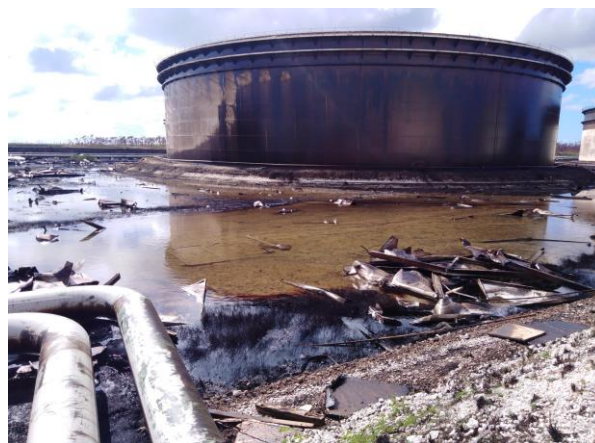
Figure 9: The containment basin around the tanks forms a closed system without drainage of rain water. This is confirmed by the presence of water and crude oil inside the basin
