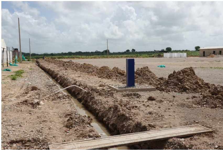
Figure 18: Ongoing expansion works at the CAI - water utilities system.
